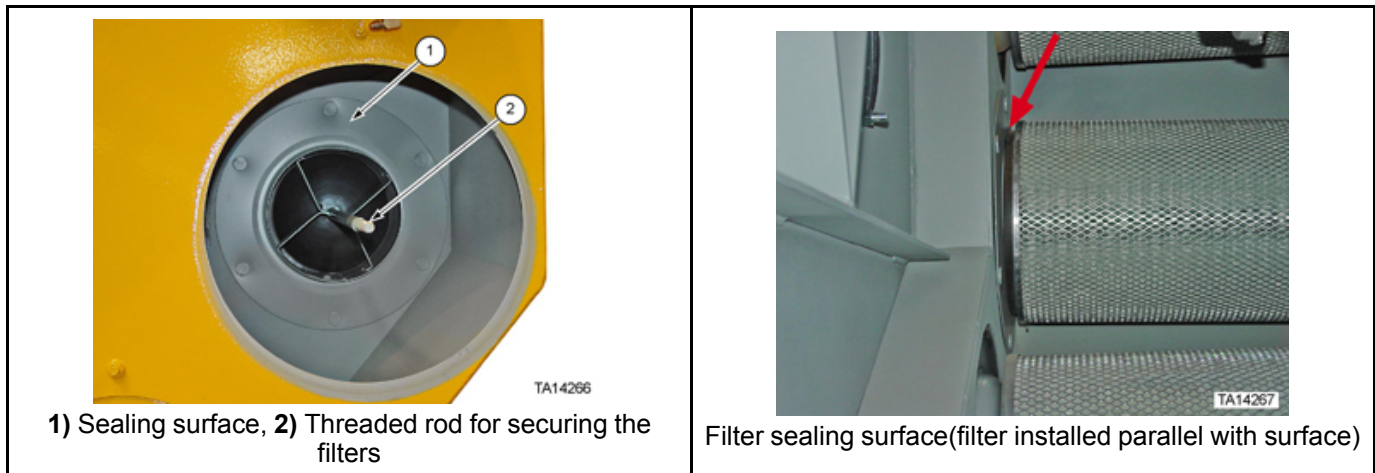
Figure 21: Filter support rod and sealing surface
