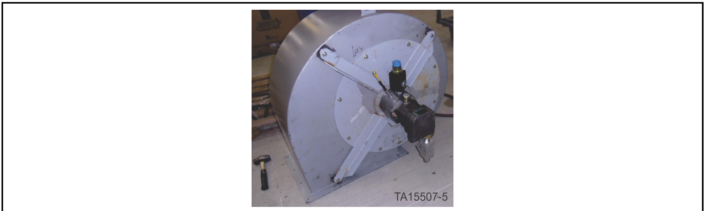
Figure 49: Blower removed and placed in work area
