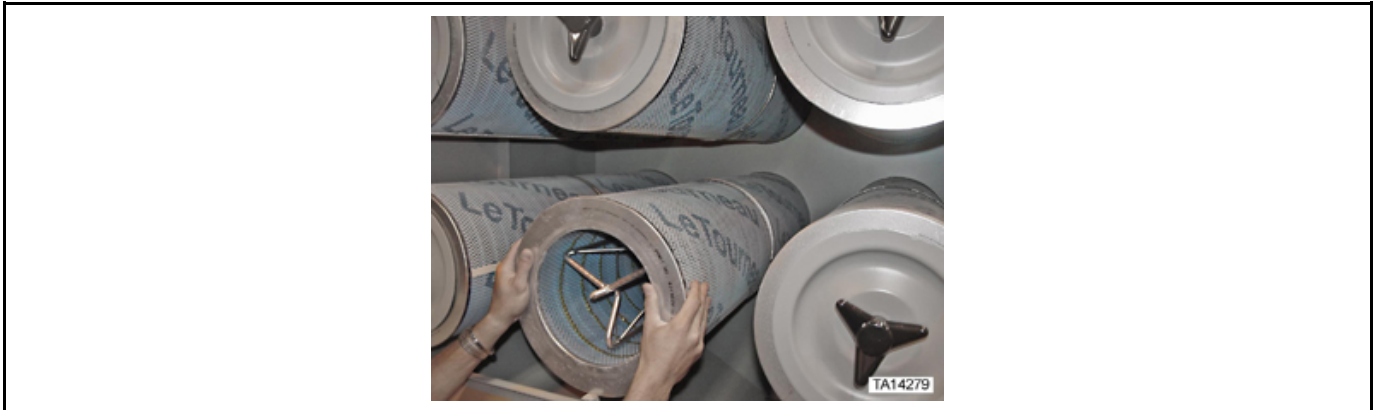
Figure 98: Removal of “KLENZ™” filters
